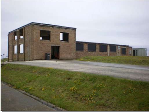
Rear of loading bay / rear of canteen
