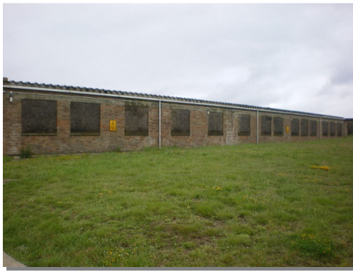
Rear of accommodation building
